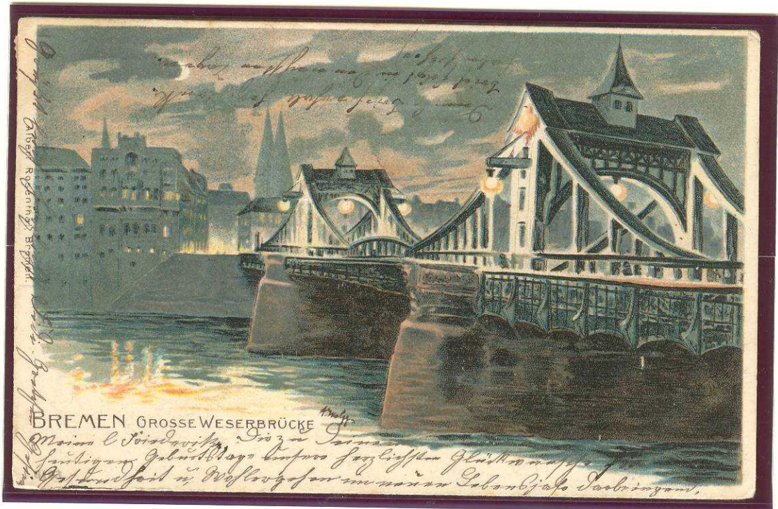
1903: Bridge Across the Weser River
